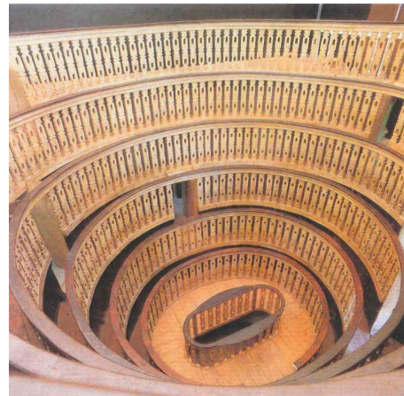
Figure 2 - Top view of the structure
