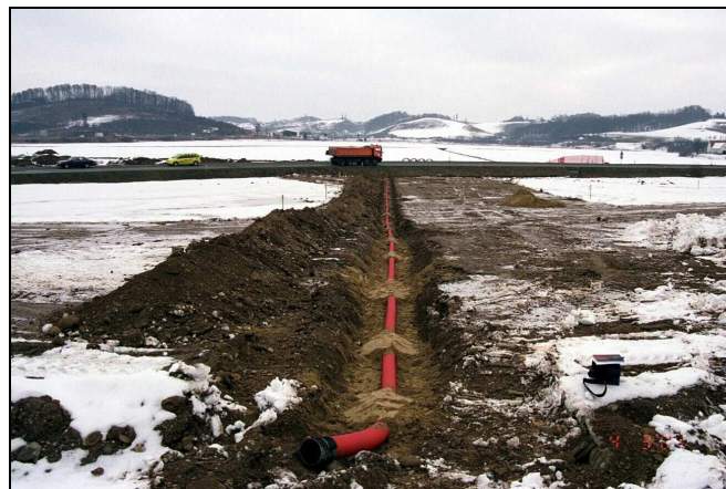
Figure 5 - Installation of the measuring tube HI-2
