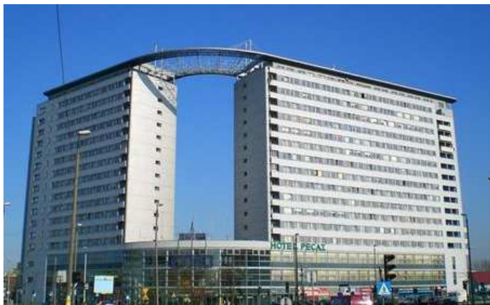
Photo. 6. Building having irregular shapes (photograph: www.panoramio.com ).
