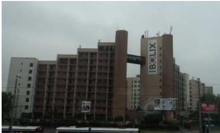
Photo. 3. Building with aboveground connector (photograph: www.panoramio.com ).
