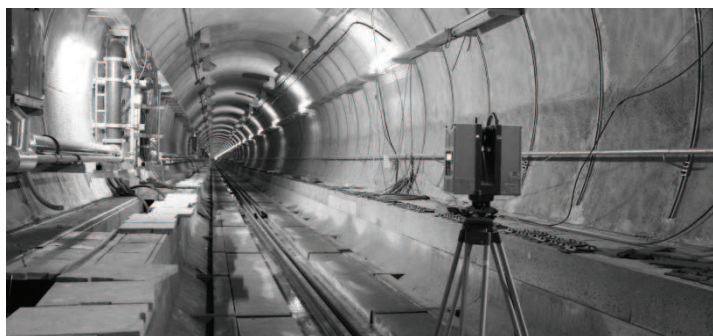
Figure 3 Laser scanner setup
