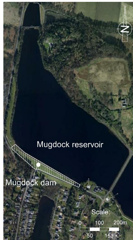
Fig. 2 Mugdock reservoir enclosed by an earth-fill dam on the south side.
