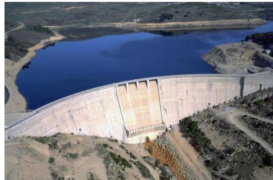
Figure 7: Aceña dam (Spain).
