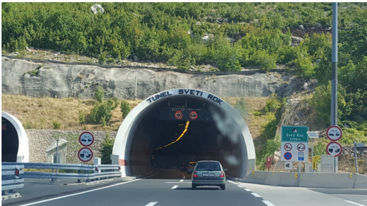
Figure 6. Road tunnel Sveti Rok
