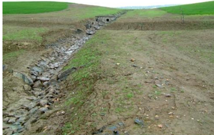
Illustration 6: Example of realization of water management measure – stabilization of concentrated runoff paths
