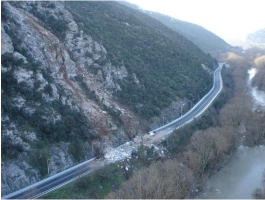
Figure 1. Tempi Valley rockfall 2009 by helicopter
