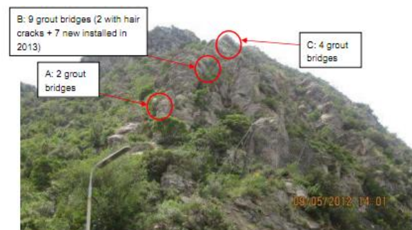
Figure 10. General View of the installed grout bridges at section 6 (old chainage 386+650).
