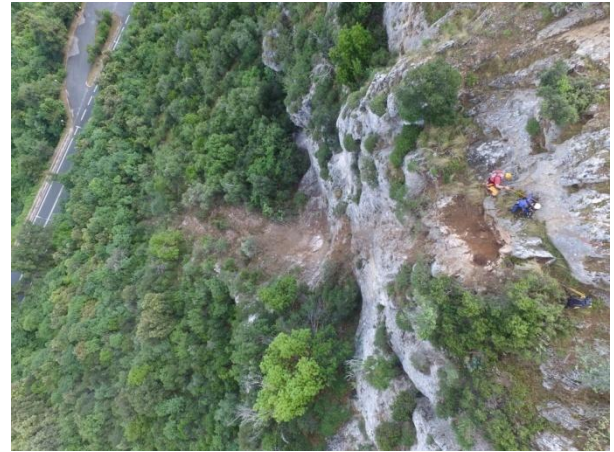
Figure 4. Inspection and scaling works
