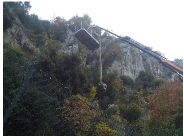
Figure 5. Emptying of barrier from trapped blocks
