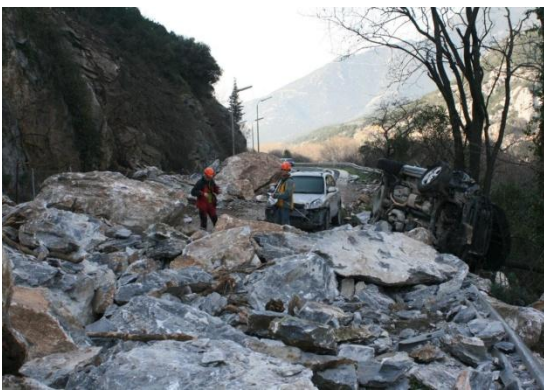
Figure 2. Tempi Valley rockfall 2009
