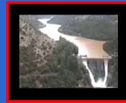
The Ladon Dam during the flooding period of February 2002. Both spillways are simultaneously in use for the first time since the hydro plant became operational in 1955.
