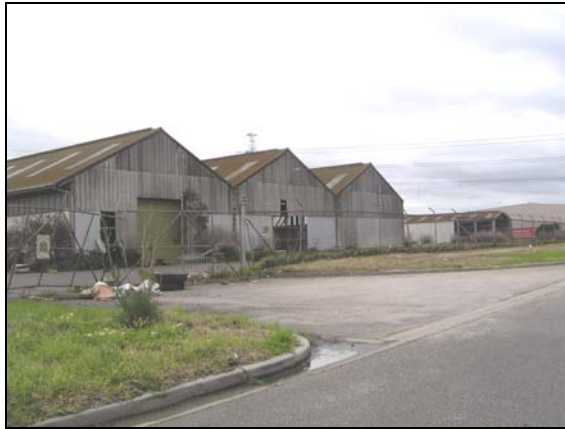
View of obsolete industrial building on the site
