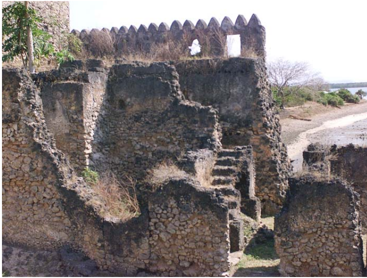
Figure 1: Broken, free standing walls inside the Gereza
