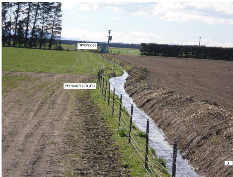
Figure 1 Effects of fault rupture on previously straight fence and water race (Photo: Survus Consultants)
