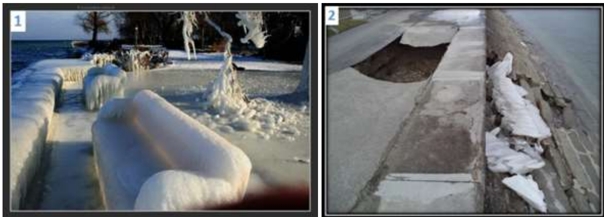
Fig. 3): Ice shield on the shore in February (left) [4]. Collapsed ground after the melting of the ice in March 2018 (right).
