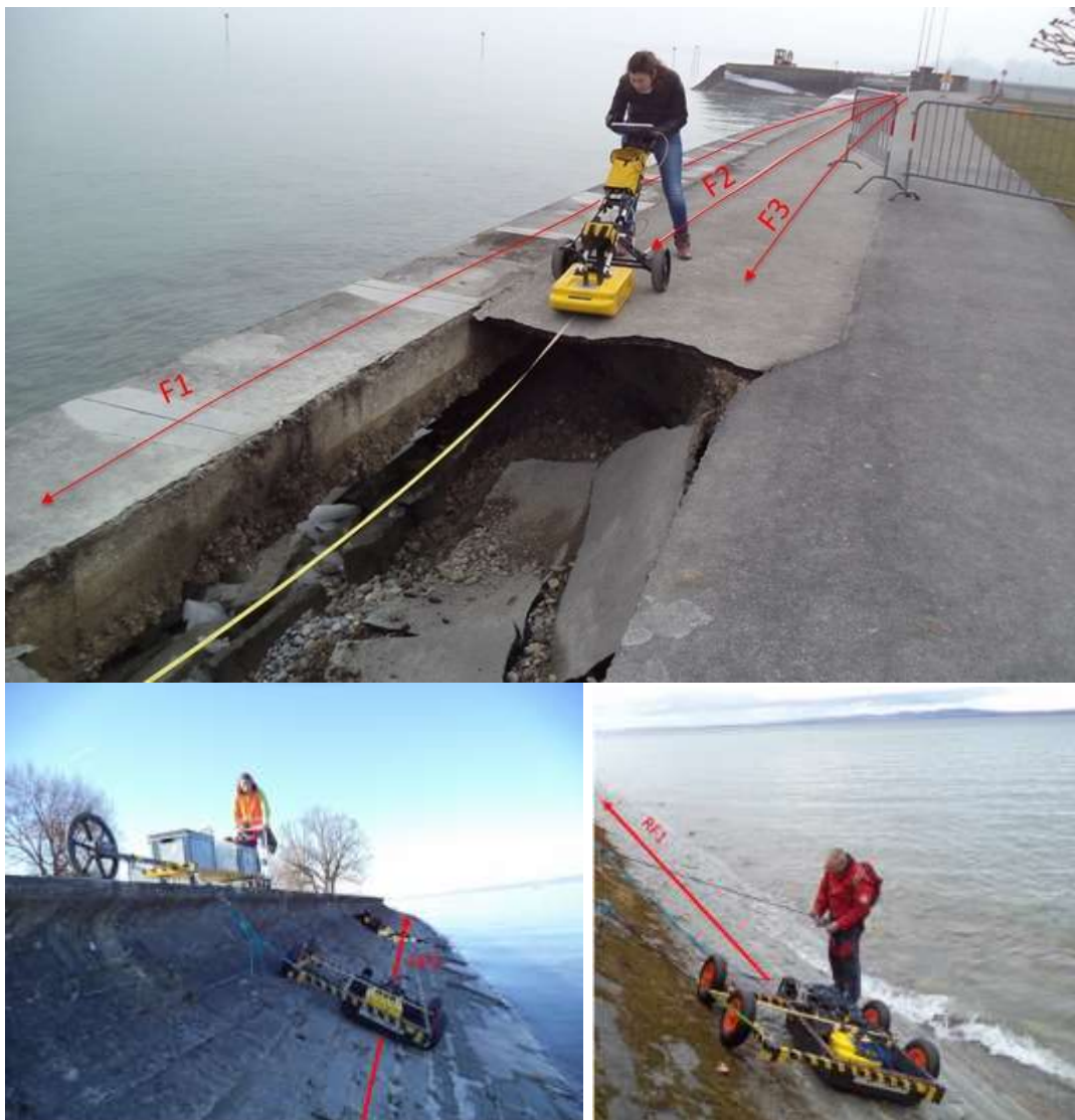
Fig. 5): GPR shots along the promenade: Three profiles on top of the path, view towards the fairground plaza (top picture), two profiles on the ramp wall, view in the opposite direction (pictures below).
