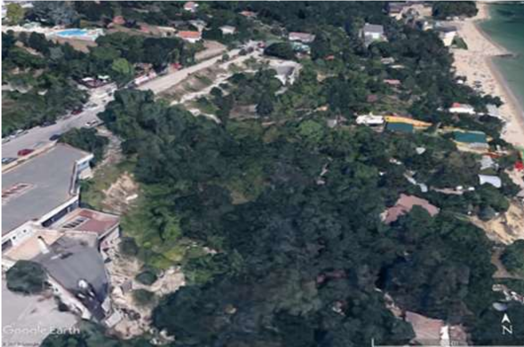
Figure 2. “Trifon Zarezan” landslide as seen in Google Earth.
