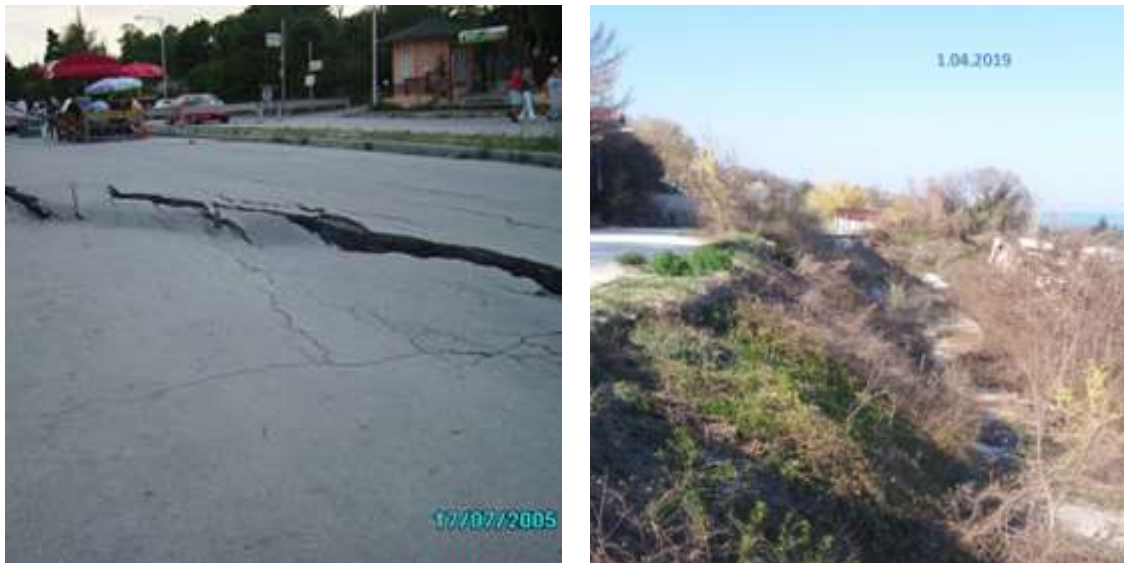
Figure 4. Cracks and subsidence in the area of Trifon Zarezan landslide
