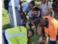
Installation of survey benchmark in Suva, Fiji. Photo by Andriak Lal
