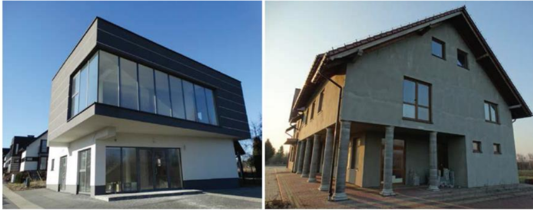
Fig. 2. Buildings with an overhang: a - without columns; b- supported by columns. (Source: Buśko M. 2016. Analysis of the influence of amendments to the legal provisions relating to building structures on keeping the real estate cadastral database updated (in Polish). Infrastruktura I Ekologia Terenów Wiejskich , 395–410)
