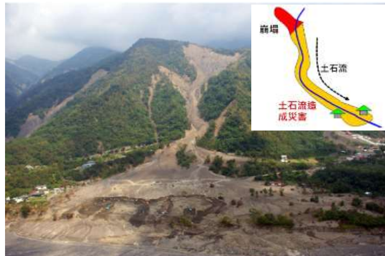
By debris flow
