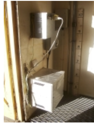
Figure 4. Receiver, power and communications housed within secure boxes.
