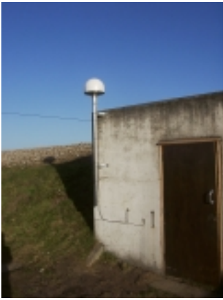
Figure 3. Antenna installation at a remote station.
