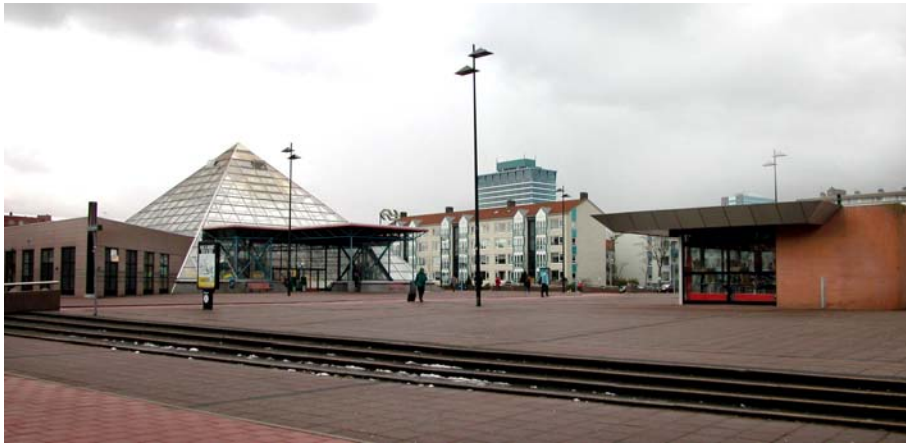
Figure 1a: Rijswijk railway station. The triangle-shaped object is the building of the railway station (parcel 7856 and 7857), the building on the right is a kiosk (parcel 7854 and 7855). The railway tunnel is located beneath the buildings.
