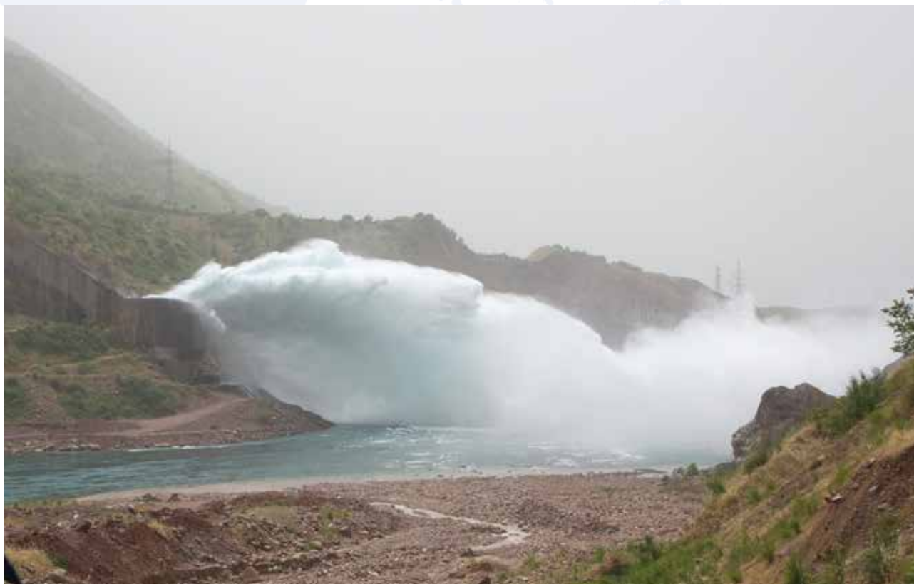
Nurek Dam and hydroelectric station in Tajikistan. Photo © United Nations/ Rick Bajornas.
