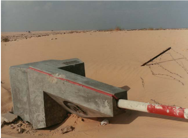
Figure 4: Situation requiring maintenance.
