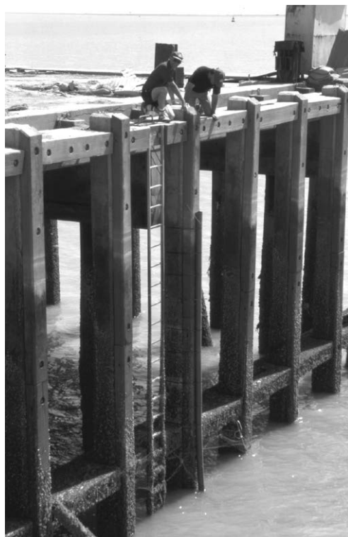
Figure 5: Installation of a tide gauge on a pier jutting into Khwar Az Zubayr.
