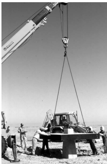
Figure 6: Installation of a pillar complex.
